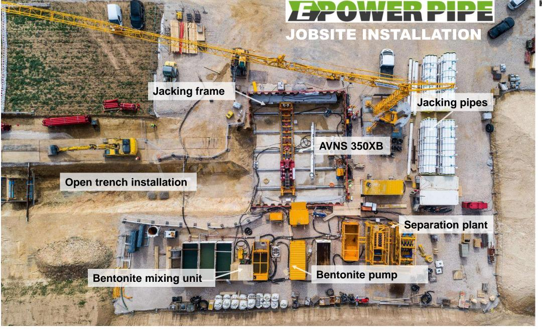
Microtunnelling assists HDD
